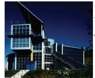
Building of the Institute of Solar Energy Research in Hameln (ISFH).
